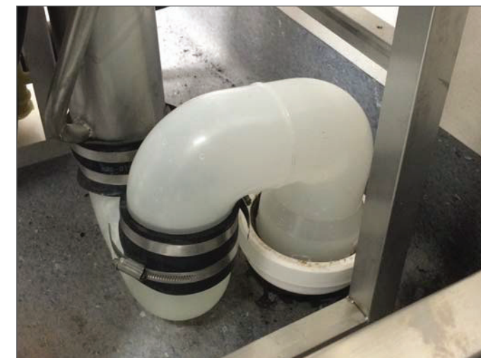
A typical drain connection pictured (above)
